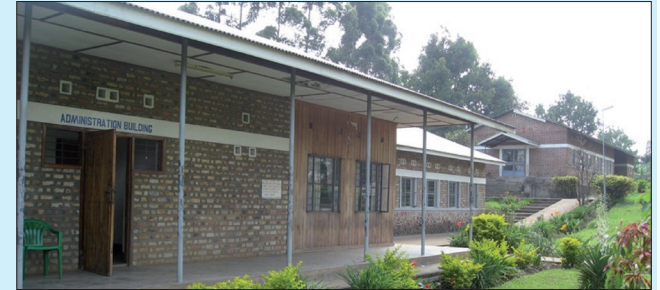
A portion of Administration Block – Kahungabunyonyi Campus
